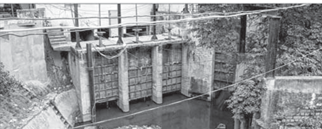
The sewage treatment plant at Bans Ghat
