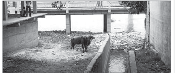
Sewage water flows into the Ganga at Anta Ghat
